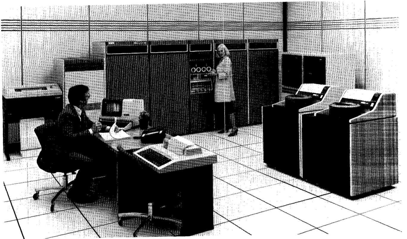
DECsystem-10s support a family of peripheral devices that includes disks, magnetic tapes, terminals and terminal interfaces, lineprinters, card readers, and a paper tape punch/reader.
