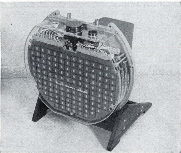
**Three subassemblies** are visible in this mockup of the computer. They are the central processor, the memory, and the input-output. The round shape is the cross section of the missile in which the computer will be used.
