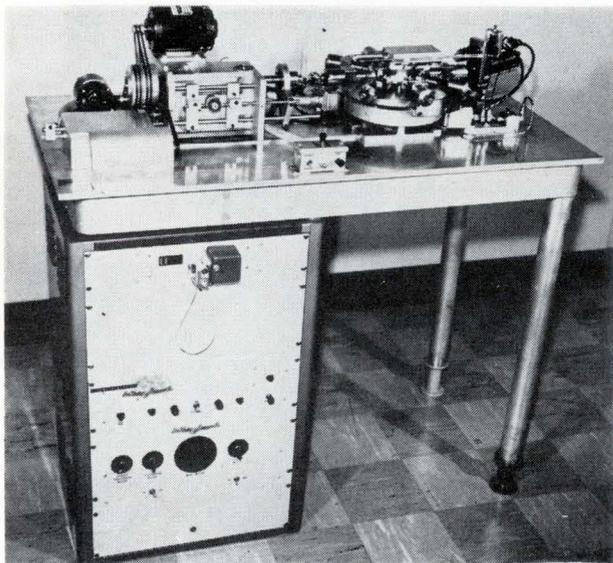
Tape control unit fits beneath a coil winding machine, and sequences any number of winding operations while controlling auxiliary assembly and test functions as well.
